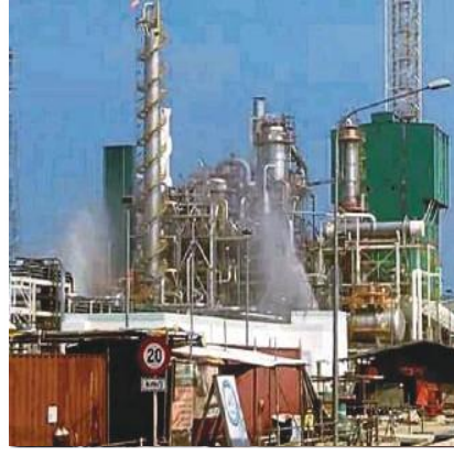
Ammonia Leak in Sabah, 2016
